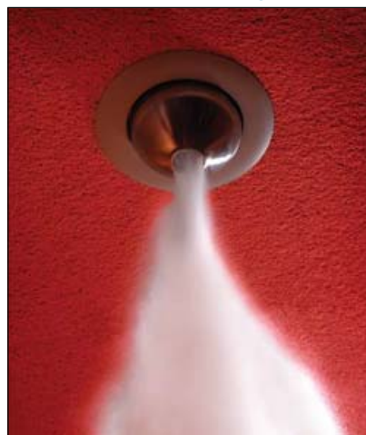
Aquasonic water-atomizing fire suppression system in operation
