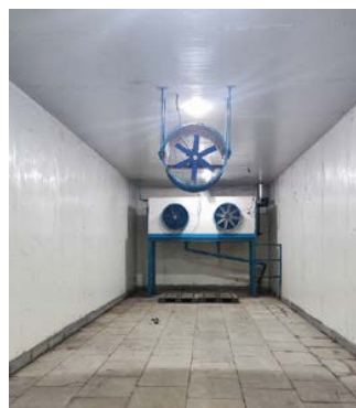
Figure 22 Indoor unit inside cold storage at site 1
