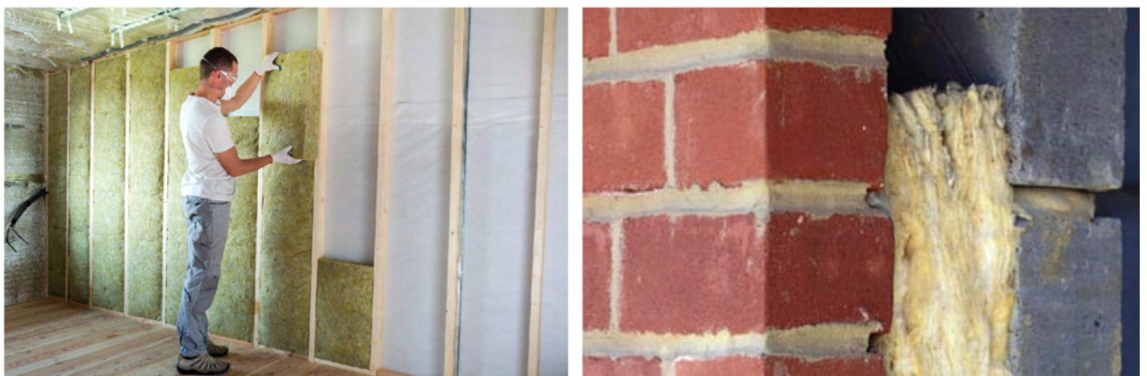
Figure 3.3 Insulation material application
