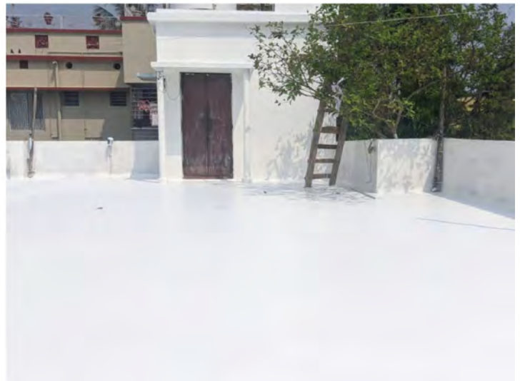
Figure 3.5: Application of reflective paints, cool roofing tiles on building roofs in India
