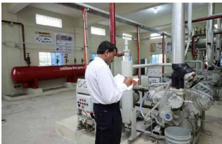
Figure 3.2: Compressor used in ammonia-based refrigerant in the cold storage system
