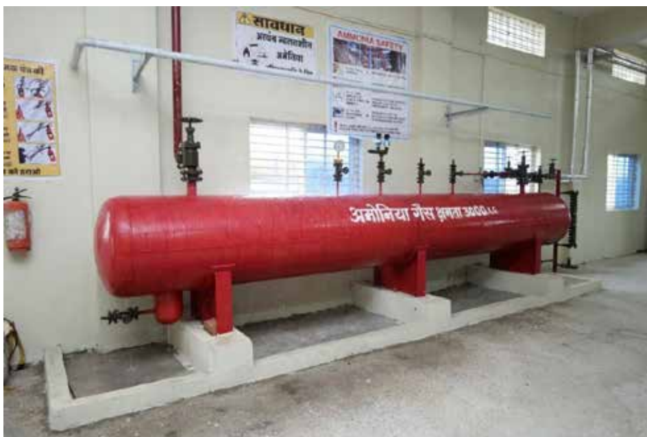
Figure 1.7: Ammonia storage facility in cold storage with all safety measures
